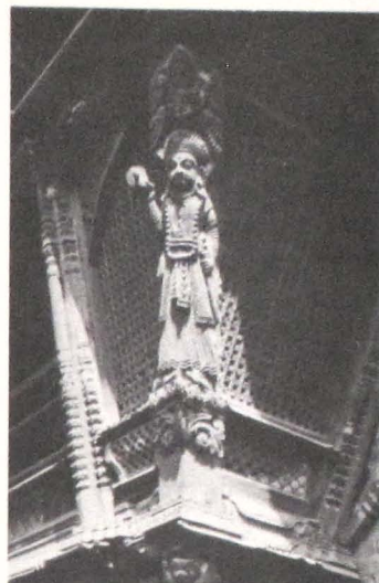
587 Bhaktapur: private house of Gvaḥmādhi, early 19th century, projecting window (sājhyaḥ) with corner strut depicting a prince with sword and pigeon.
