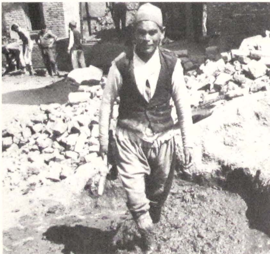
347 Helpers (cākaḥmi) knead the clay with their feet before it is used as mortar.
