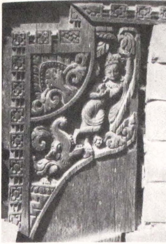
622 Wall bracket (gvāḡaḡkva) of Hariśaṅkara temple in Taumādhi / Bhaktapur.
