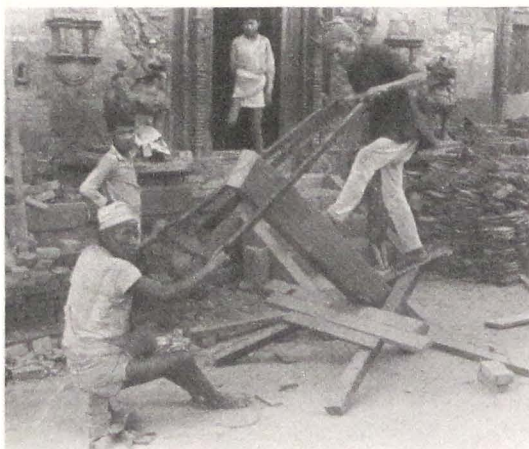
639 Carpenters (sikaḥmi), cutting a log into boards with a bucksaw (bvasikaḥti).
