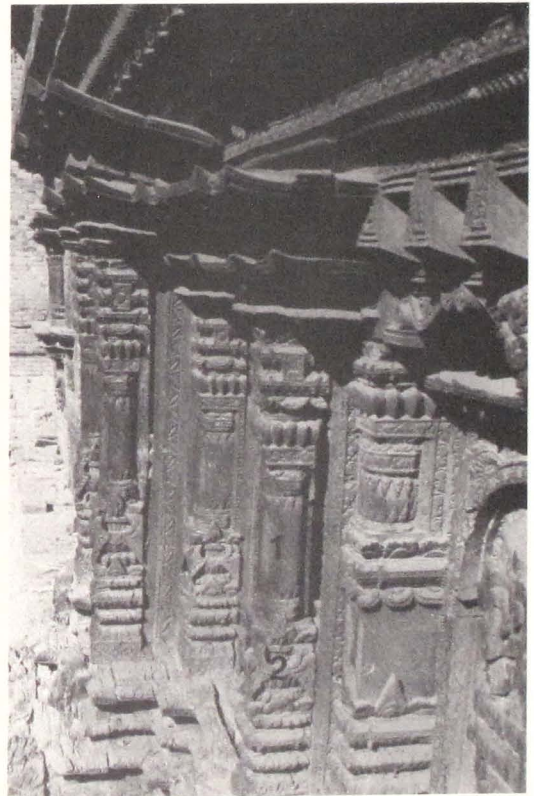
575 17th cent. pasukājhyāh with 'classical' tvalāthā: a base with kalasa design (2), an undecorated middle part (1), and a capital with prominent āsa design.
