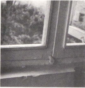
543 Closing pin (hāytvaḥ) of a modern window.
