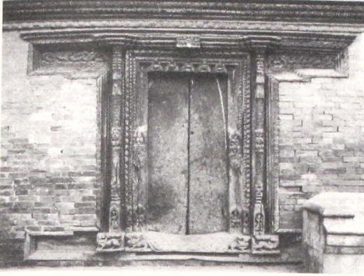
508 Pāṭan: Sundarīcuka (courtyard), 1627. Secondary threshold (kvagā) in front of the jambs and individual bases under the tvalāthā-pillars.
