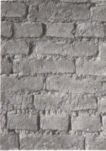
348 Wall with unbaked bricks (kaciapā) using headers every fifth layer.
