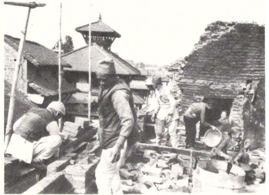
346 Bricks are washed (usually by female members of the household) before being used for construction.
