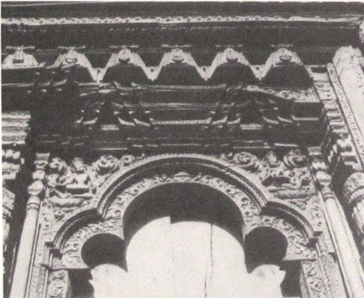
591 Gokarṇa: Gokarṇeśvara, 16th cent., tertiary lintel with kulā-design, placed below the lintel (mūtāgāh) and above the cusped arch of the door opening.
