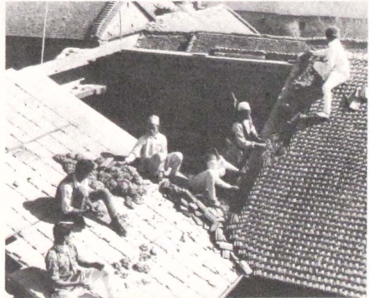
254 Roofing: placing clay (dācā) onto the lower roof tiles.
