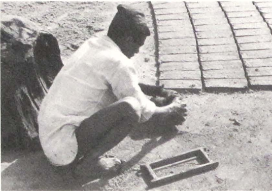
290–292 Casting of lower roof riles (cilāy).
