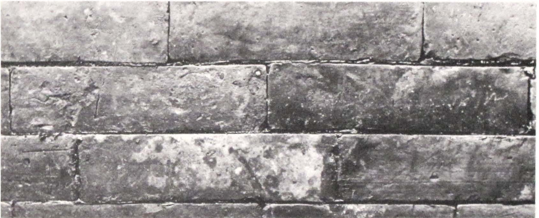
317a Surface of a wall with conical bricks (dātiapā), producing flush joints.
