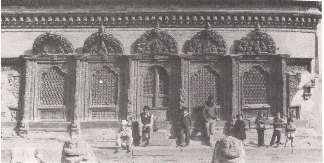
515 Kāthmānḍu: Navayoginī degah, c. 1790. The only known portal with 5 screened openings, 4 of which are reduced to windows with apron screens.
