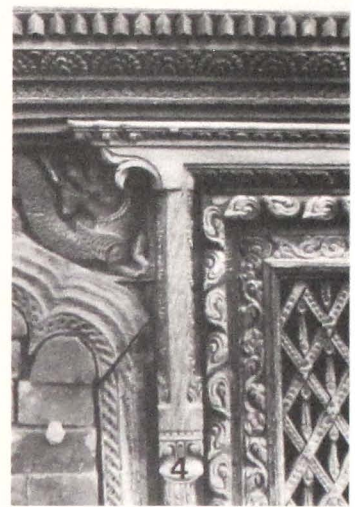
573 Together with lintels, 19th cent. tvalāthā are portal-like, the post ending in capitals of cypress design.
