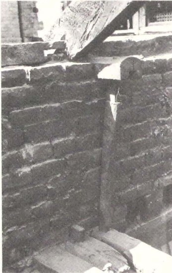
264 Jamb wall (gaḥkū) from inside with cross-tie (baigāhkāh), wall plate (baigāhṣi) and long wooden peg (cukū).
