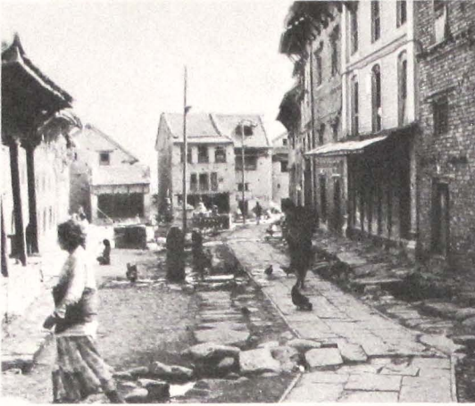
30 Balābu: a path leading to the major shrine of the settlement is paved with dressed square stones (lvahā). The drains (dhaḥ) on either side of the path are covered with longish boulders, and the rest of the surface is left as it is.
