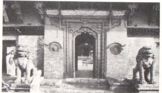
512 Pāṭan: Darbār, northern wing, 19th century. Kisidhvākhā – elephant gate with small door leaf – macākhāpā (or kacakhāpā).
