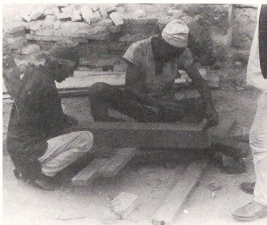
640 Carpenter (sikaḥmi), marking the cutting lines with a thread (hākhi).
