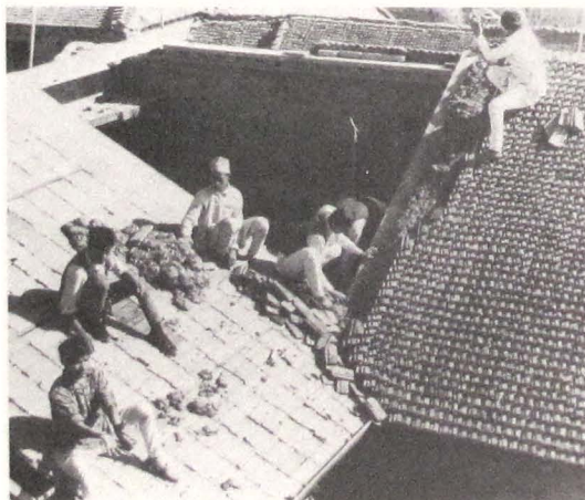
641 Roofer (āvāh), placing mud mortar onto the lower roof tiles.
