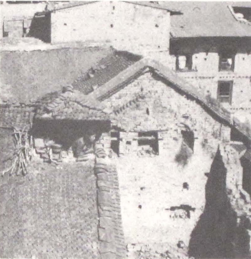
270 Dormer on ridge level.
